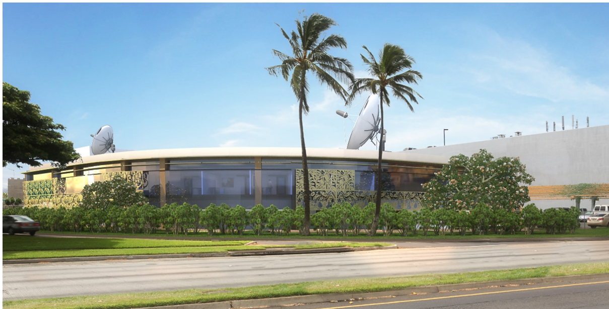
Construction on PBS Hawaii's NEW HOME on Nimitz Highway and Sand Island Access Road is slated to begin before year's end.
